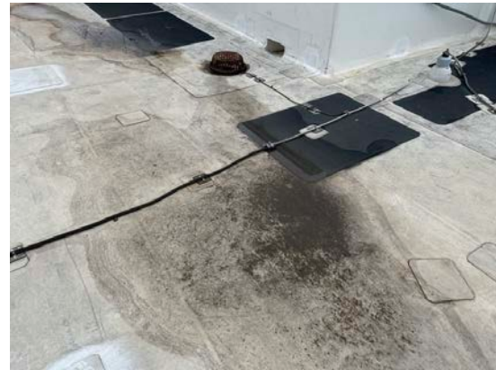
Roof-Area of Concern
