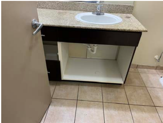
Bathroom Lavatory - Unit 12006
