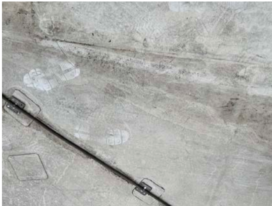
Roof-Area of Concern
