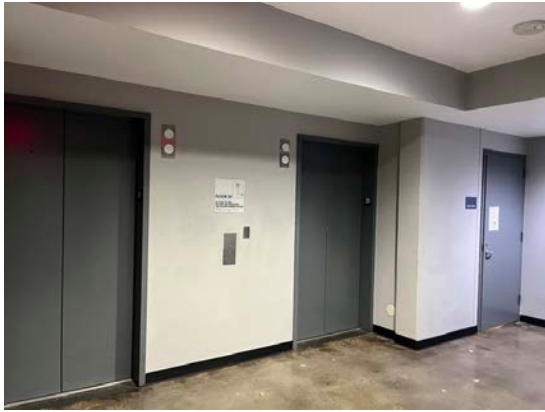
20th Floor Elevators
