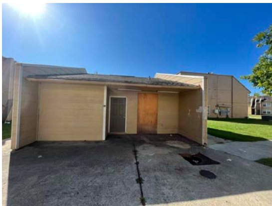
Community Laundry Facility Exterior
