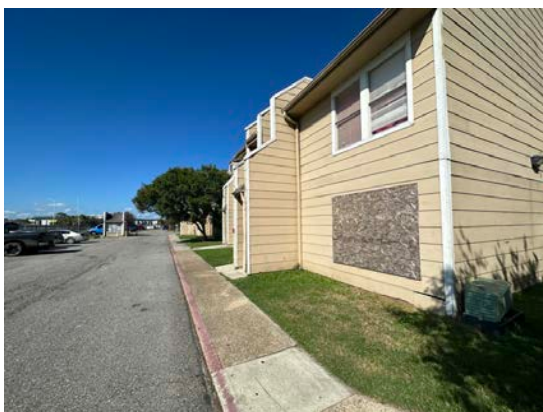
Subject Property Partial South Elevation
