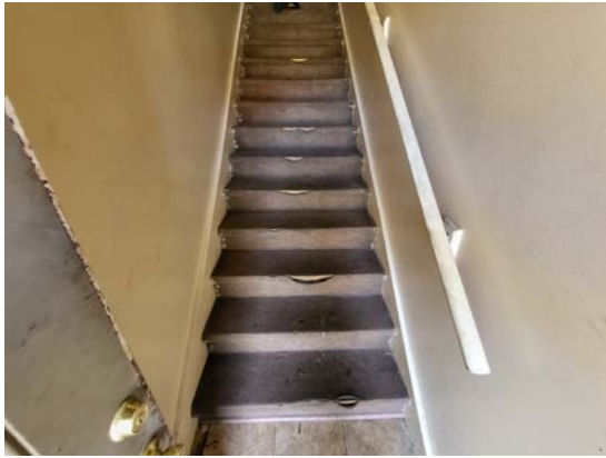
Stairwell to Units
