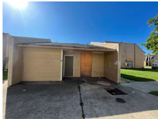
Community Laundry Facility Exterior
