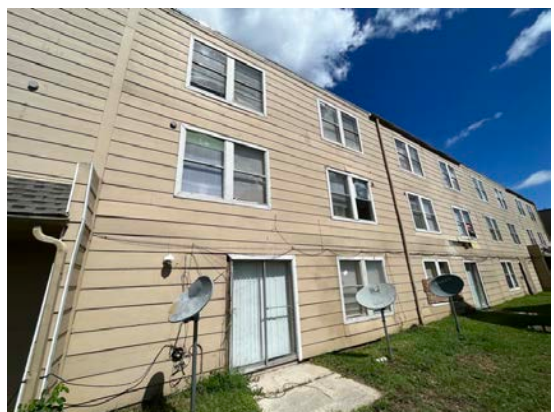
Apartment Building Exterior
